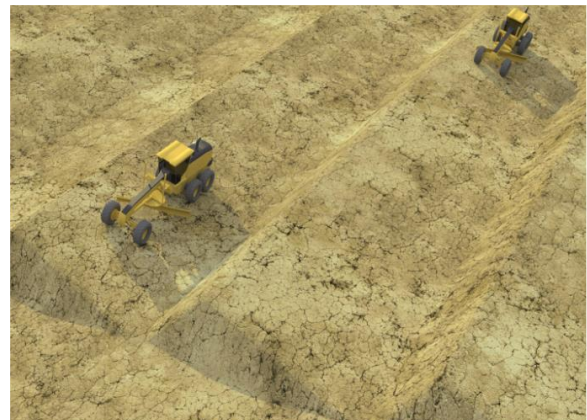
Figure 8: Earthmoving for north-south slopes construction.
