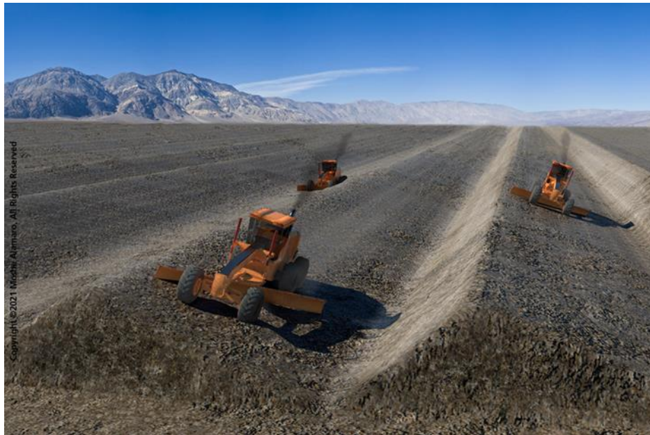
Fig. 1: Earthmoving by graders for slope construction
